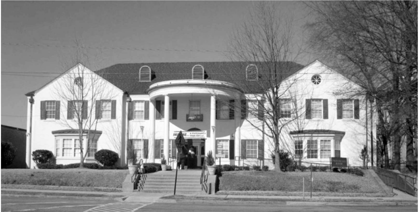
Providence House was originally a Victorian mansion, but was remodeled in the 1930s into the Colonial Revival style.
