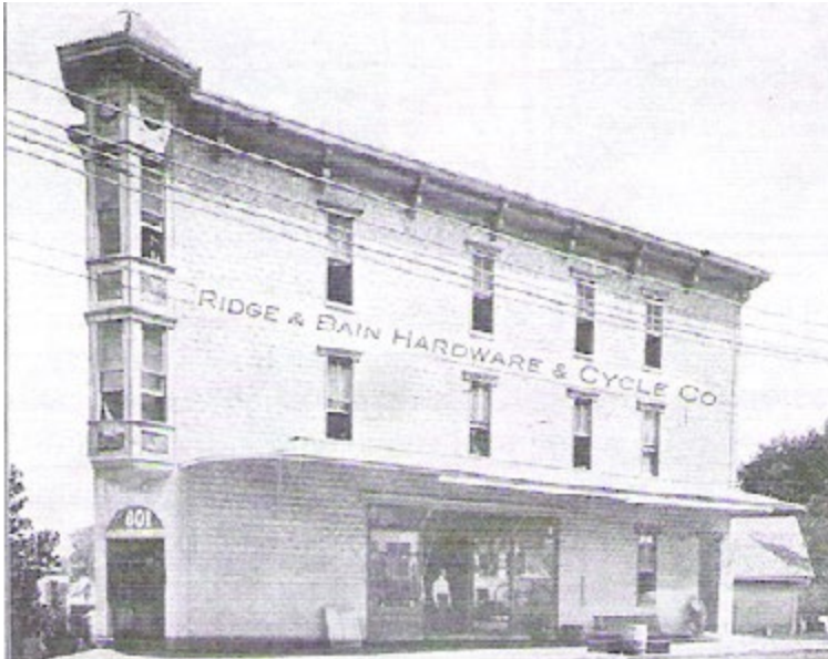
This triangular wood frame Italianate style building was built between c. 1900 at 801 Texas Avenue. It was an early mixed-use facility with two hotel floors above its commercial storefront.
